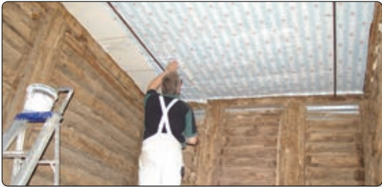
Installation of ceiling wallpaper in entrance of Kow Plains Homestead 2011
