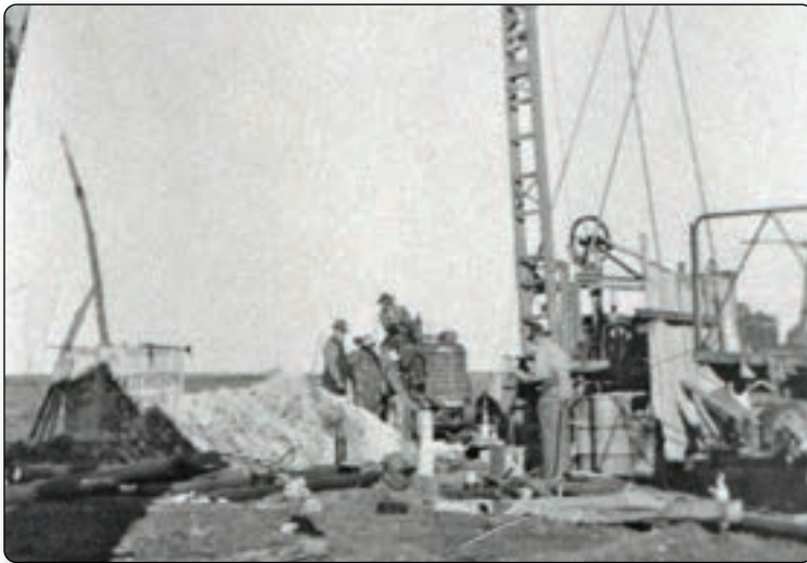
R. Forsyth drilling a bore for water at Tutye, 1958, for irrigation
