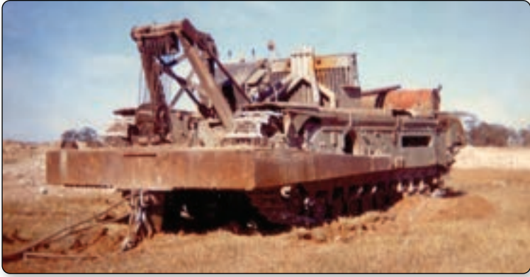
Ripper used to rip stone after blasting Kow Plains Quarry late 1960s
